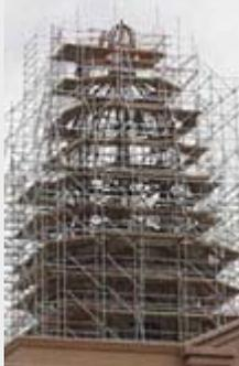
The clock tower of a historic 1895 Texas courthouse has been stripped to its steel skeleton as construction crews restore the deteriorating top hat of Fort Worth's most distinctive building. The 1940s-era clock, which will be in a protective box until the dome is re-covered, will keep on ticking rather than be replaced with a digital mechanism and will still require manual resetting when
