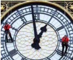
Workers for British height-safety specialists TaskMasters recently rappelled down the clock faces (each 23 ft. in diameter) of the tower that houses Big Ben to find and repair damage to the glass panels.
